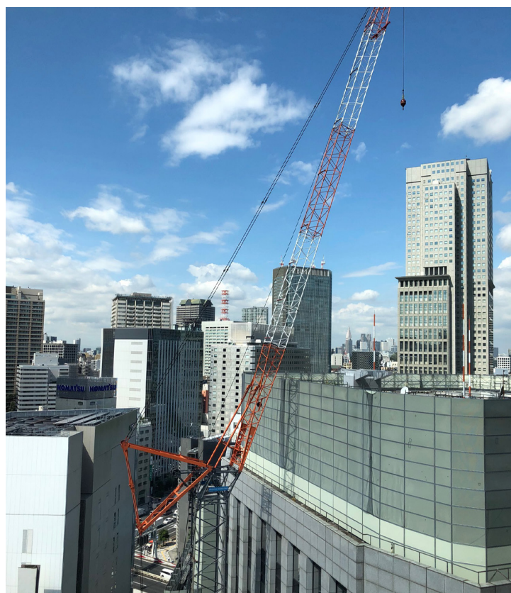
Blue skies for construction work around Tokyo. Source: S&P Global Platts
